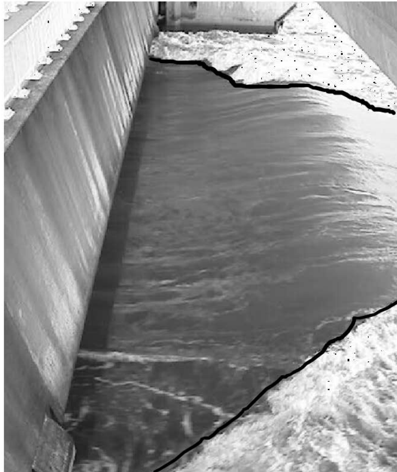
Fig. 1. Oosterschelde storm surge barrier.
