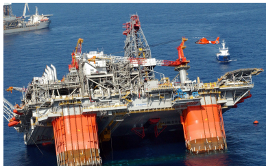
(e) Offshore oil platform “Thunder Horse” tilted by hurricane Dennis.
